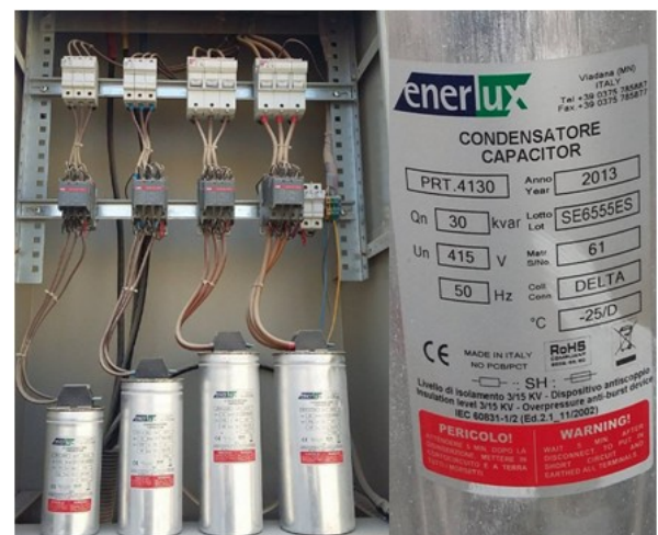
Fig 4.7 delta capacitor bank connected in transformer.
