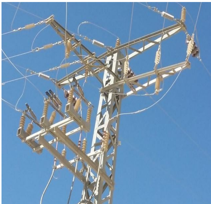
Fig 5.4: Isolator is not clean and dirty.
